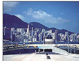
Western Harbour Tunnel (WHT)
