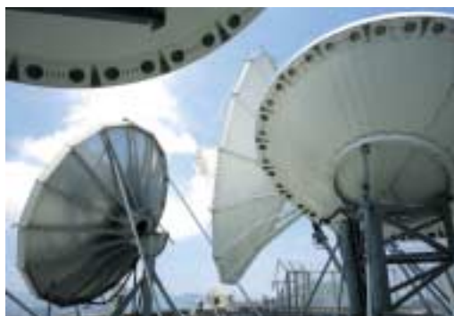
Cable TV Tower
