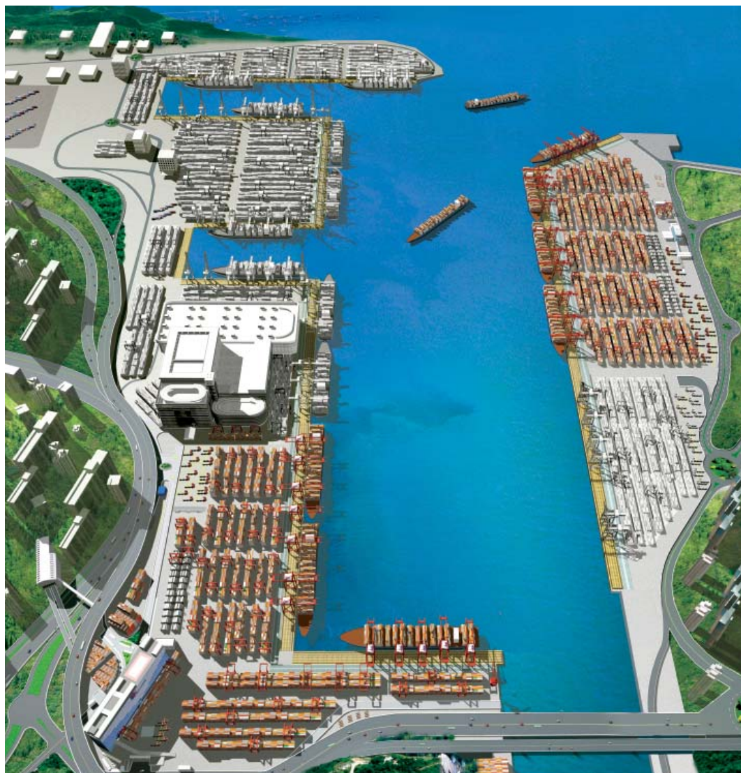
Modern Terminals' operations in Kwai Chung will consist of 7 1/2 berths, spread over Container Terminals 1, 2, 5 and 9, by the fourth quarter of 2004.
